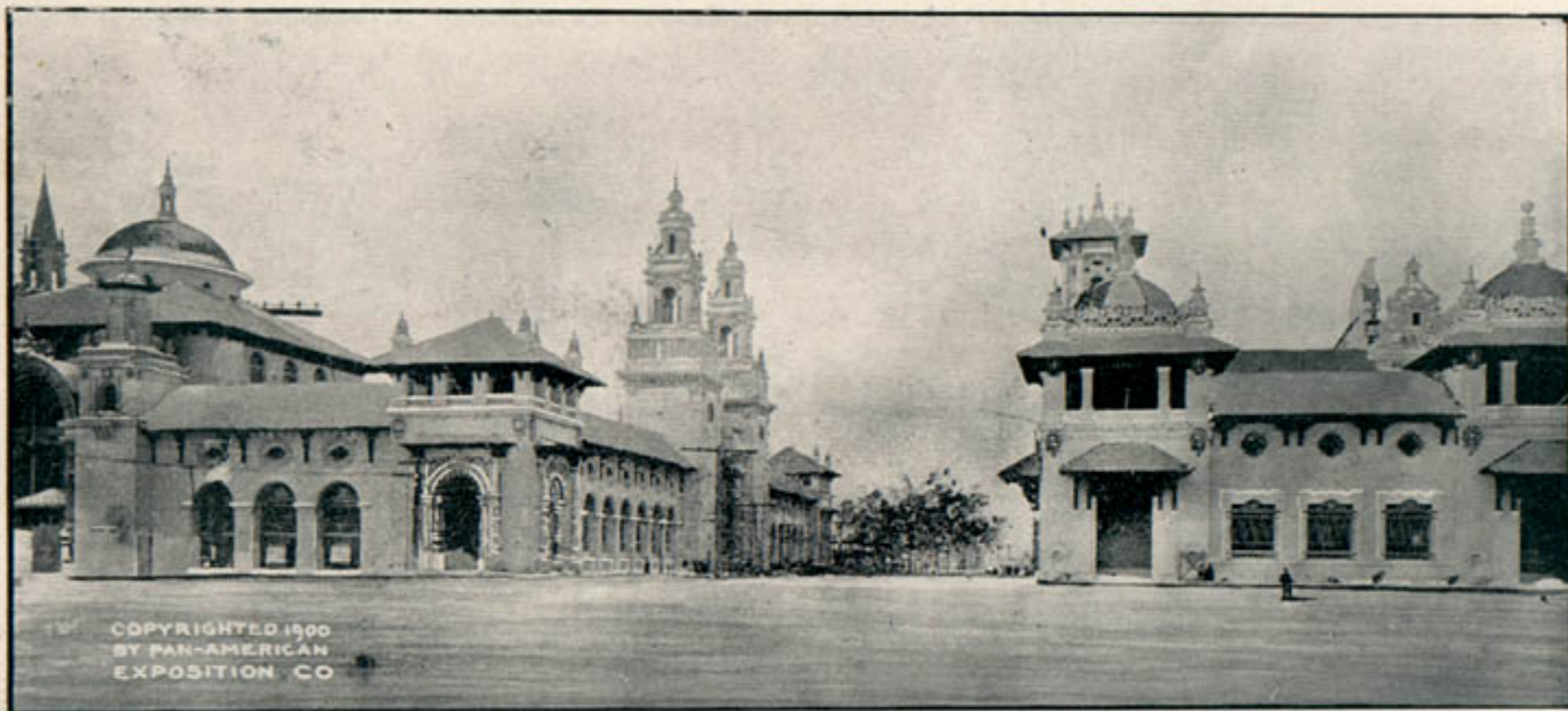
MACHINERY, TRANSPORTATION AND ELECTRICITY BUILDINGS.
